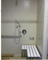
The CBC calls for hand-held sprayer mounting bracket to be mounted no higher than 48" AFF to the top. The top bracket of the sliding bar as shown on the diagram to the left appears to be 12" to 18" above the 48" max., putting the hand-held spray out of reach to a wheelchair user if a previous standing user leaves it in the high position. Providing a second shower head in lieu of a sliding bar as shown in this picture would meet the intent of the code.
