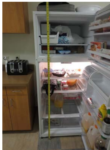
Access specialist verifies work surface maximum height of 34” AFF, unobstructed side maximum high reach of 48” AFF and maximum depth of 10” to appliances’ operable parts. A maximum depth of 24” is allowed when the side maximum high reach is 46” AFF.
