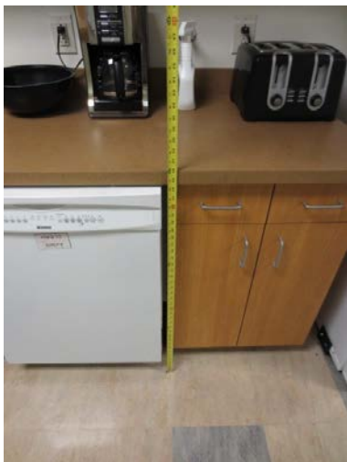
Access specialist verifies work surface maximum height of 34” AFF, unobstructed side maximum high reach of 48” AFF and maximum depth of 10” to appliances’ operable parts. A maximum depth of 24” is allowed when the side maximum high reach is 46” AFF.
