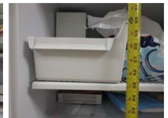
Access specialist verifies that at least 50% of refrigerator/ freezer space is at a maximum of 54” AFF. In some cases, side by side refrigerators are specified during design to ensure compliance.
